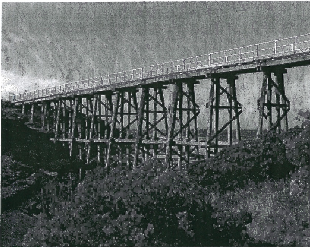
Former Kilcunda Rail Bridge
