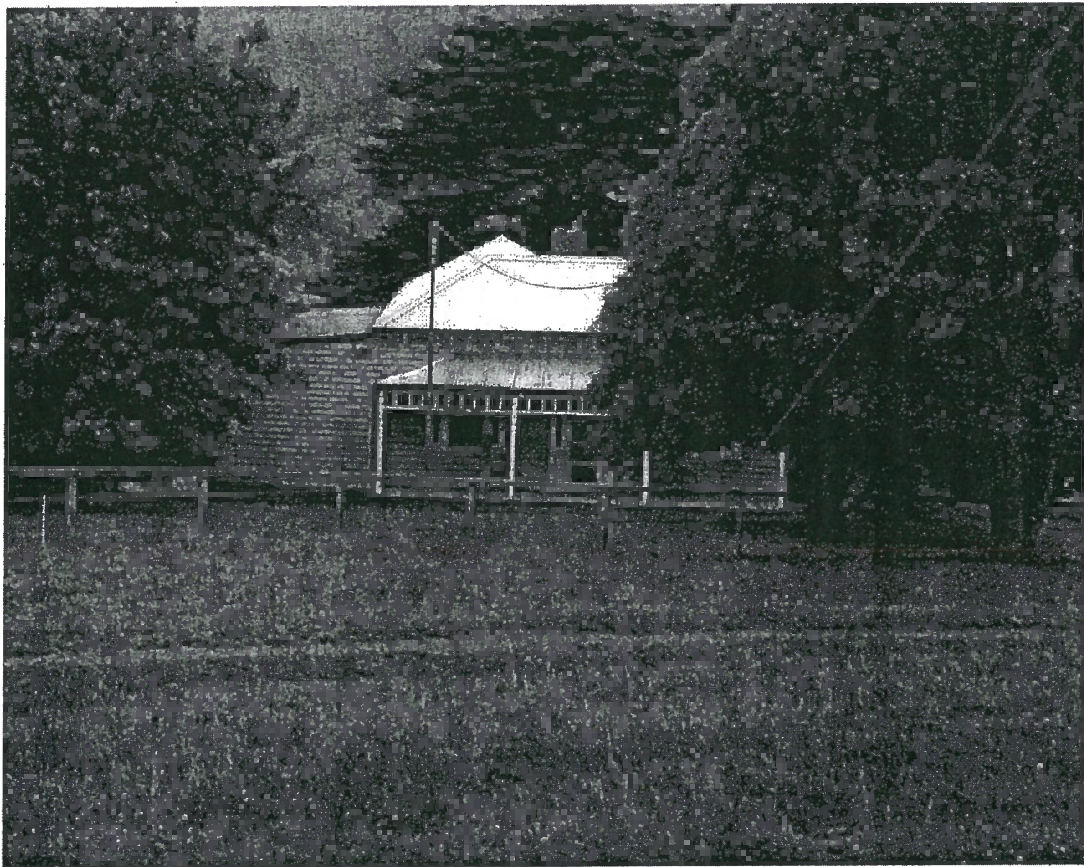
'The Cottage', 1135 Loch-Wonthaggi Road, Krowera.
