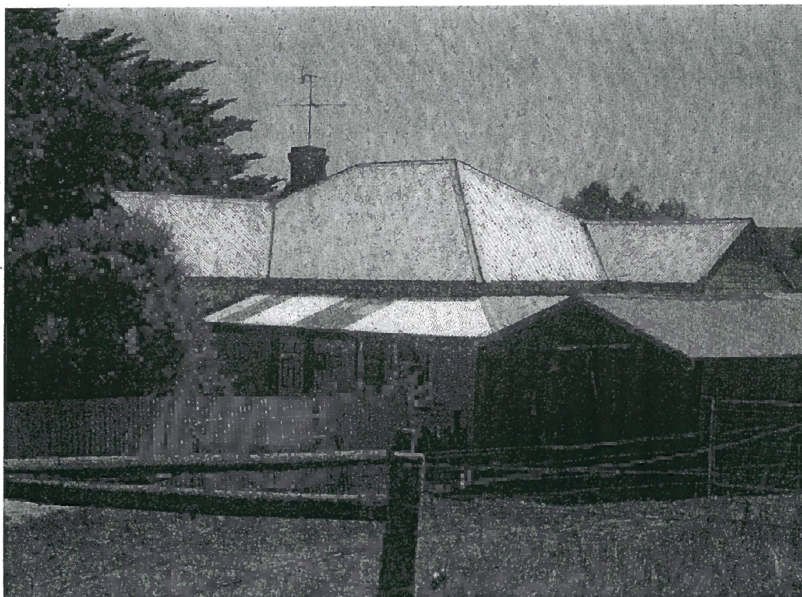
House, 55 Michie Road, Krowera
