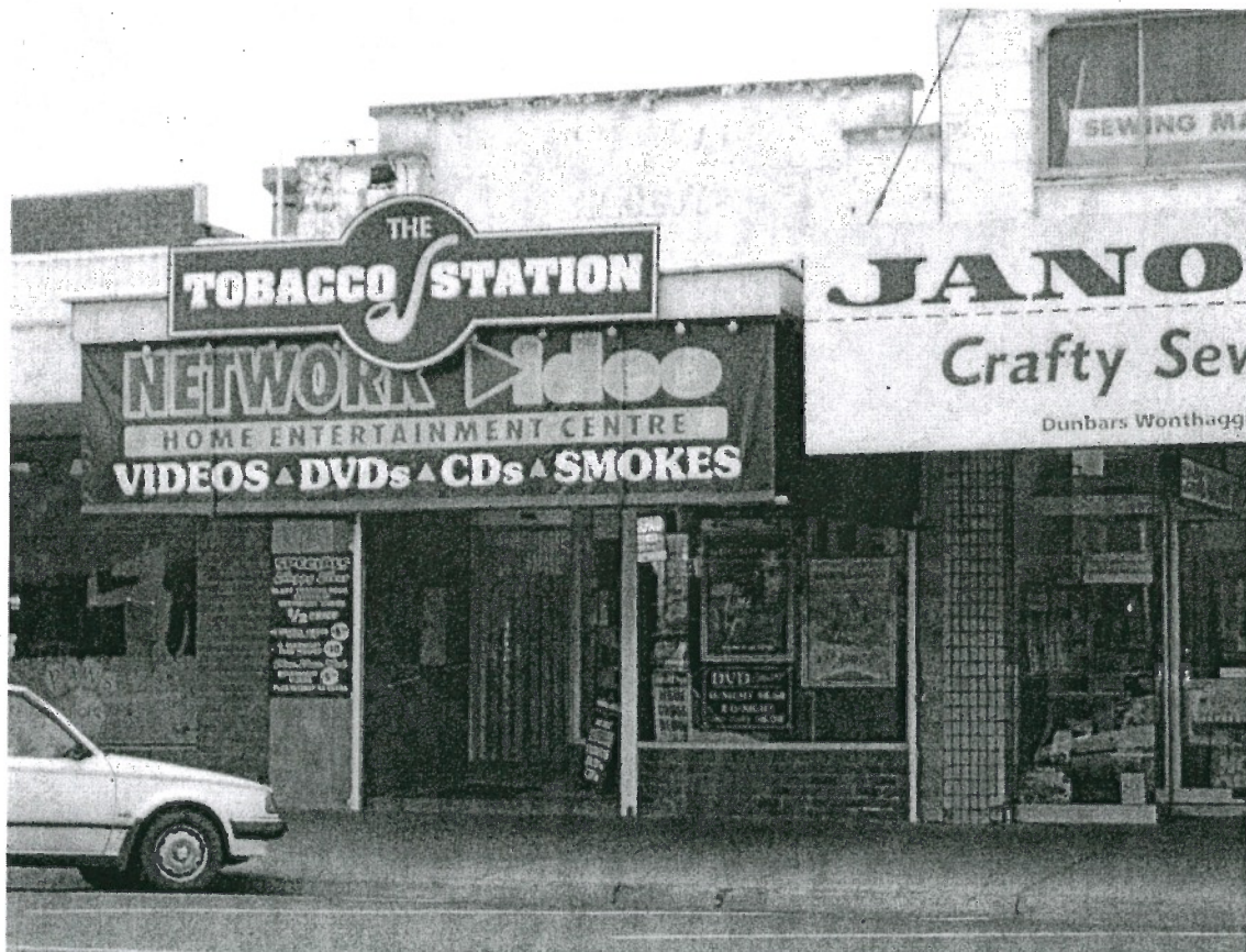
Shop, 165 Graham Street, Wonthaggi
