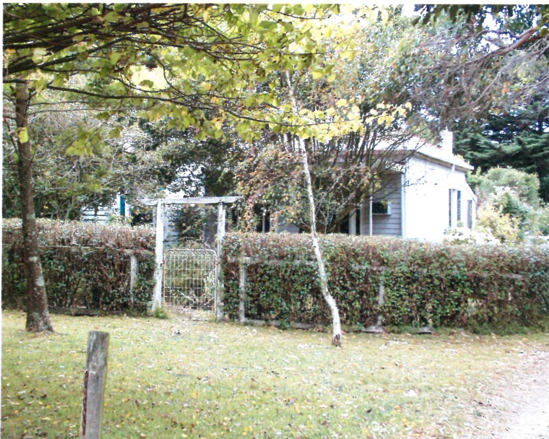
'Merricourt', 1715 Loch-Wonthaggi Road, Blackwood Forest
