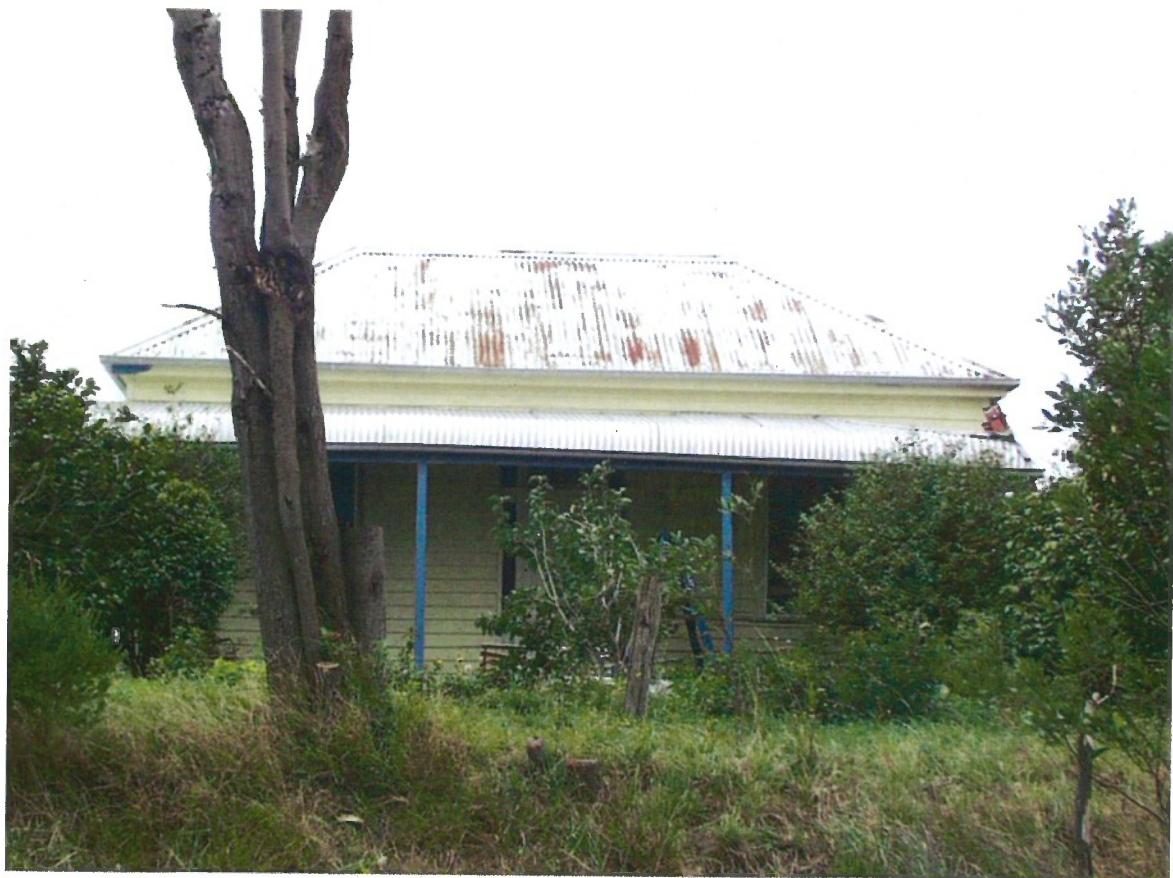
House, 1827 Loch-Wonthaggi Road, Blackwood Forest
