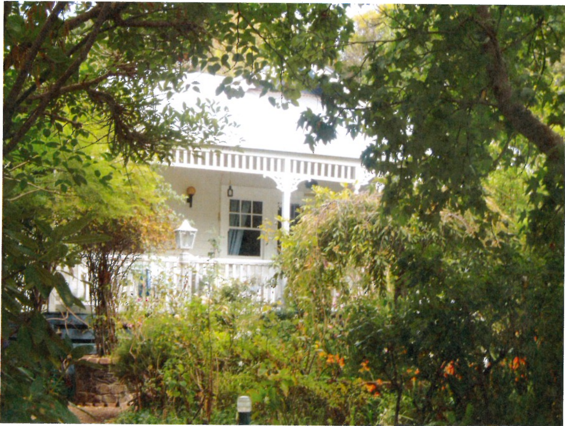
House, 16 Steele Street, Cowes.
