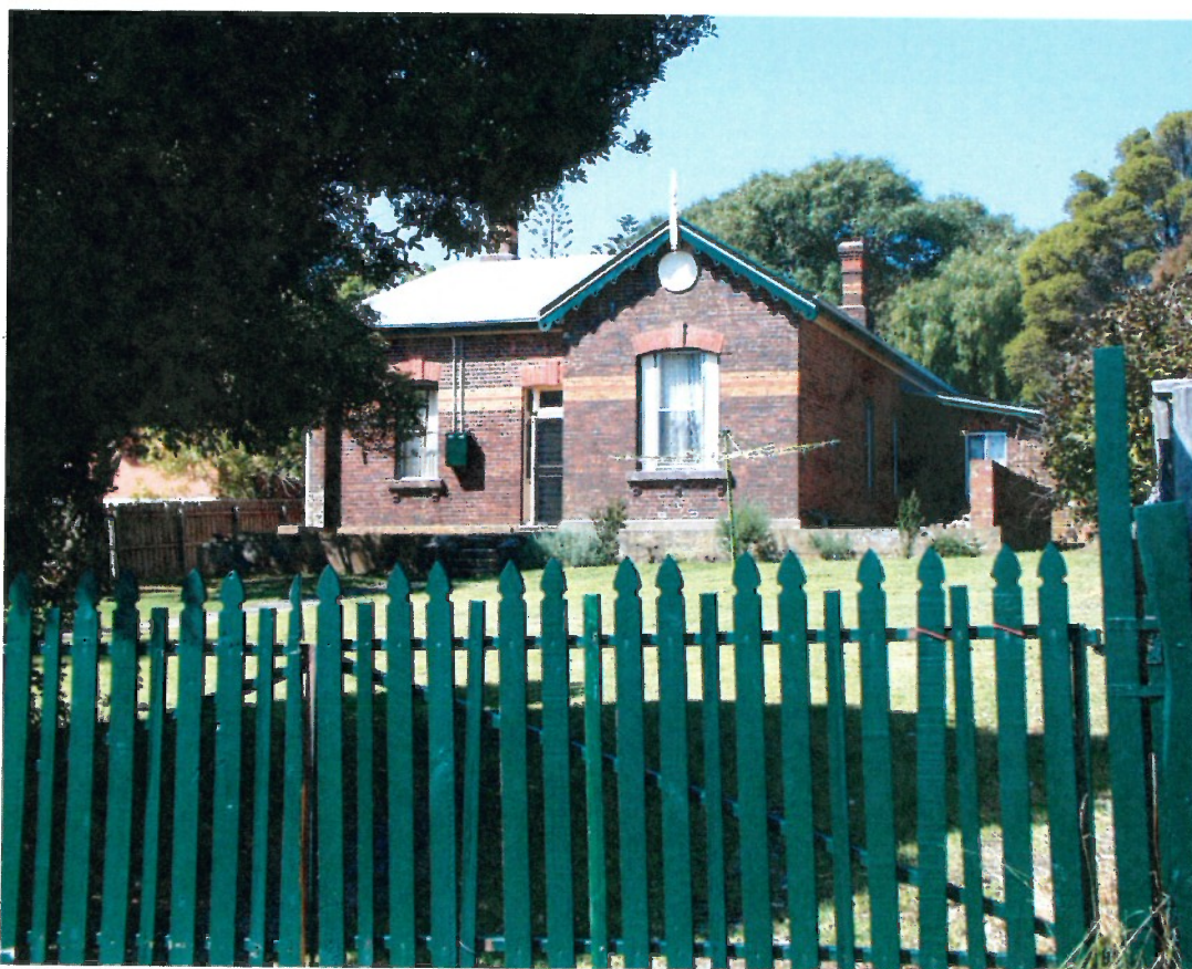
House, 11 Walpole Avenue, Cowes
