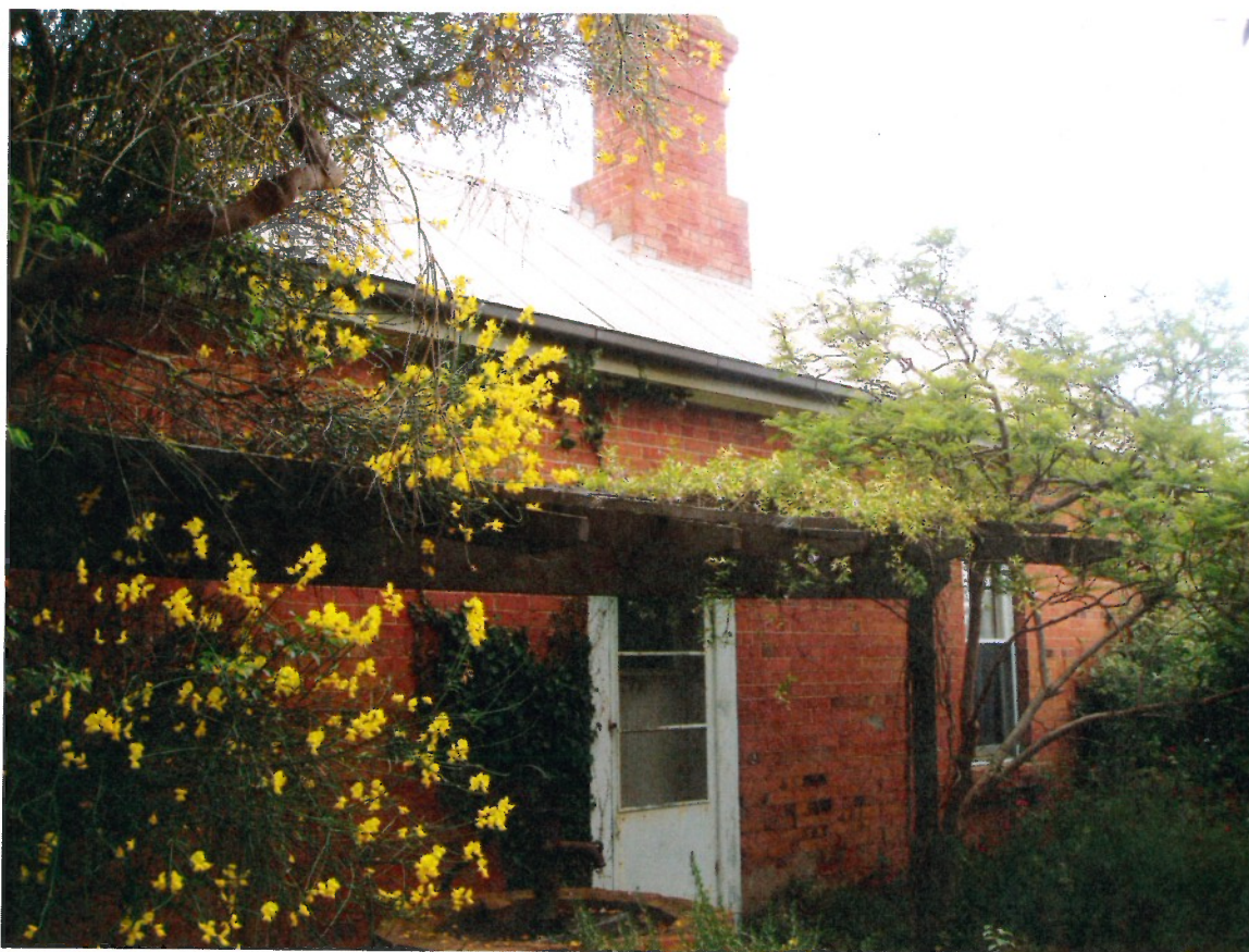
House, 13 Walpole Avenue, Cowes.
