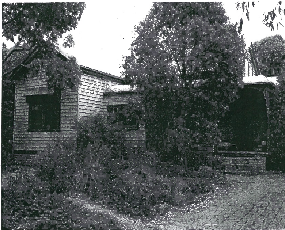
House, 37 Pier Road, Inverloch
