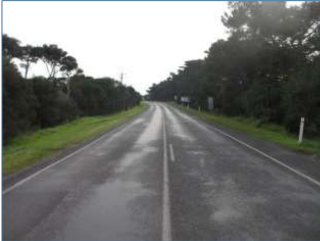
Figure 6: Cape Paterson Rd – View North
