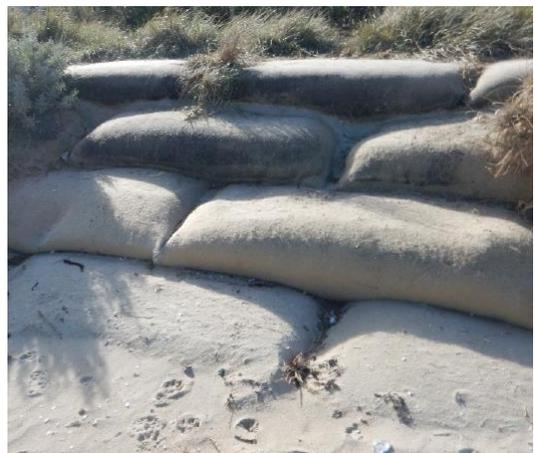
Image: Example of a sand-filled geotextile container wall
