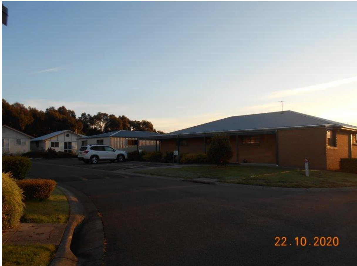
Photo 6: Looking north-east toward the existing recreation buildings and visitor car parking
