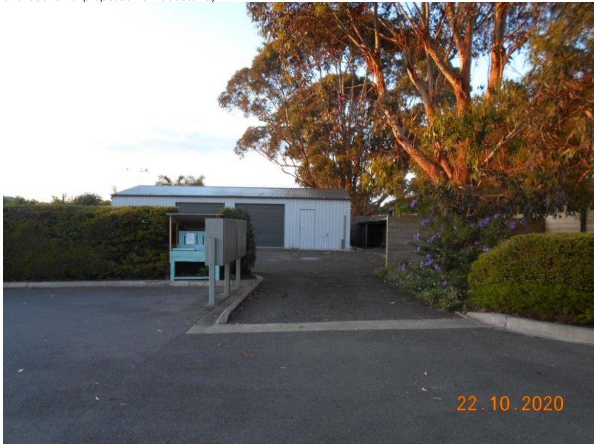
Photo 2: Looking south from the site entry, toward the shed that is to be removed
